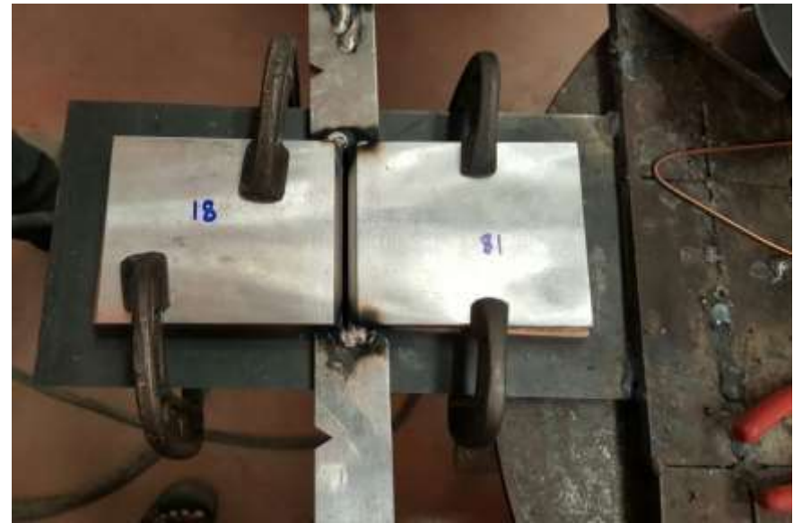
Fig: Mounting and clamping of weld plates
